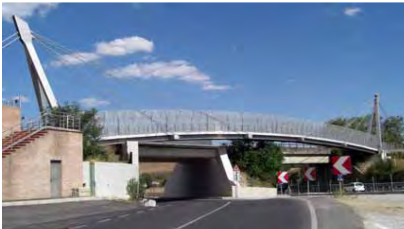
Figure 3: Highway view of the completed bridge
