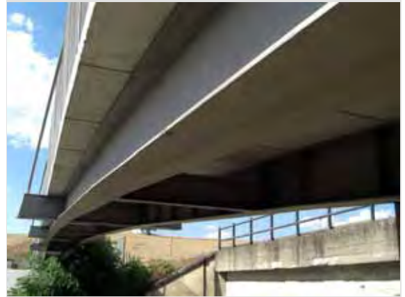
Figure 2: Underside of bridge, showing longitudinal and transverse beams supporting the deck
