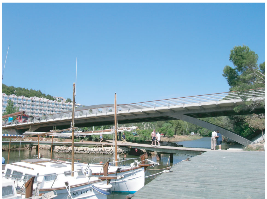
Fig. 1: General view of the bridge over Algendar river
