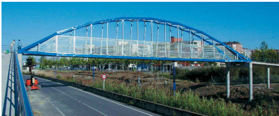
Fig. 1: General view of the entire GFRP footbridge
