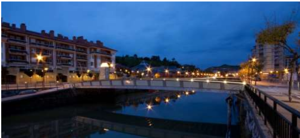
Figure 4. Zumaia pedestrian bridge.
