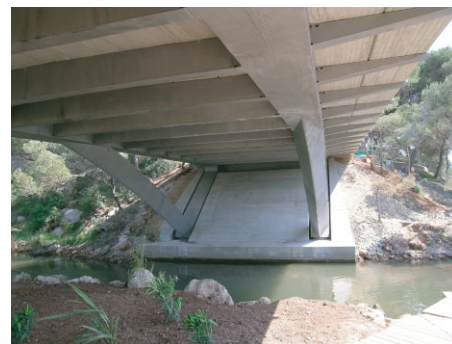
Fig. 2: Abutment 2. view of the completed element
