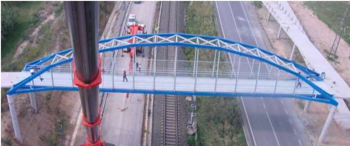
Figure 3. Lleida GFRP pedestrian bridge.
