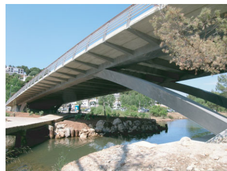
Fig. 4: View of bridge from below
