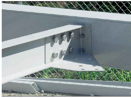
Fig. 6: Connections between floor profiles
