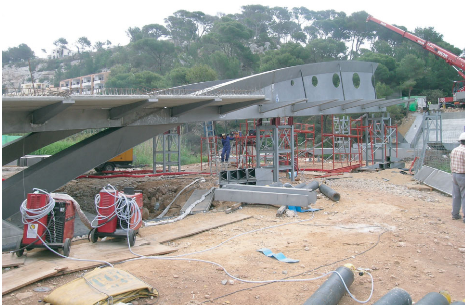
Fig. 8: Assembly of the steel structure
