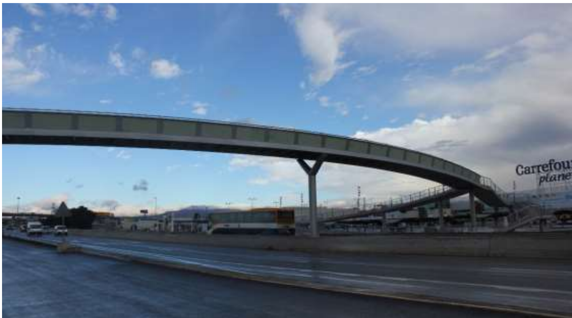
Figure 7. T-11 pedestrian bridges.
