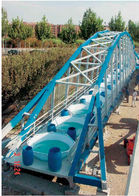
Fig. 9: General view of the load static test made before the final erection of the bridge
