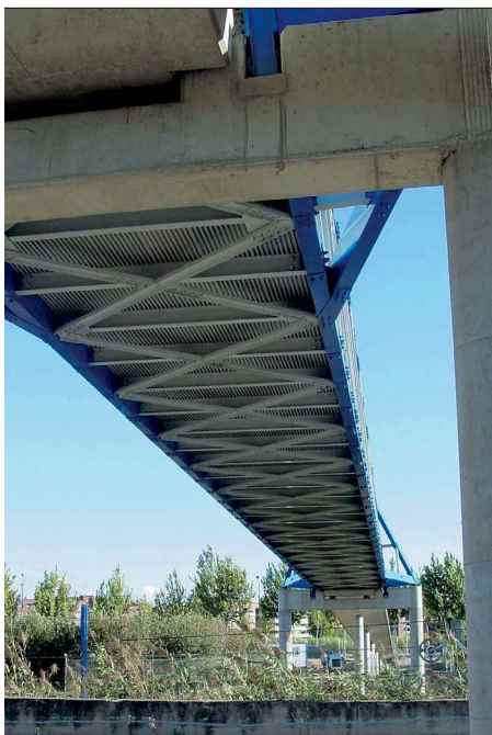
Fig. 5: Floor system
