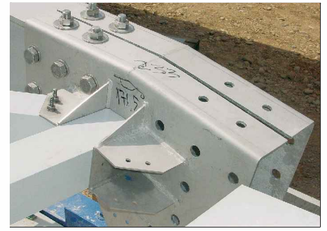
Fig. 7: Connections in the arch
