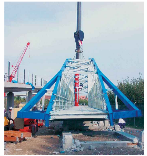
Fig. 10: Erection of the bridge
