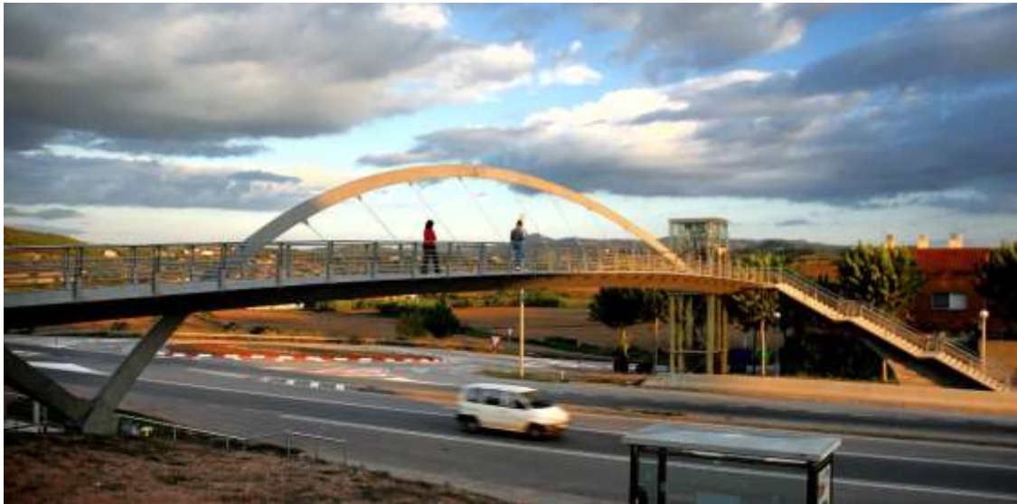
Figure 2. Sant Fruitos pedestrian bridge.
