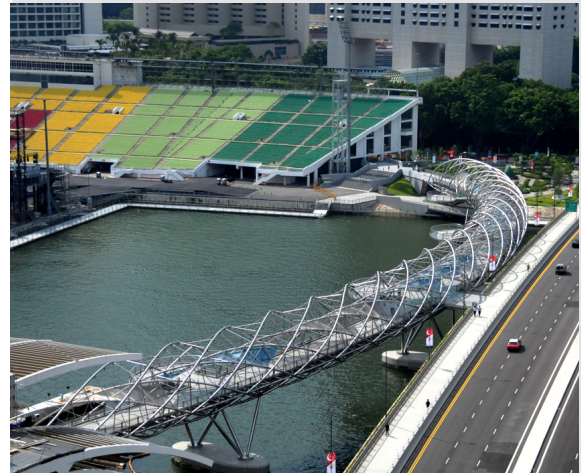
Figure 8: Finished bridge in service (Photo: Mah Guan Pang)
