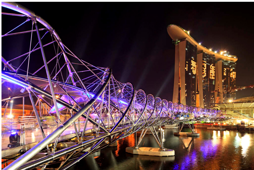
Figure 1: General view of the Helix Bridge
