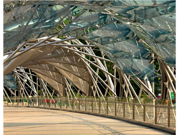
Figure 3: Pedestrian view through the bridge, including shelter panels (Photo: Arup)
