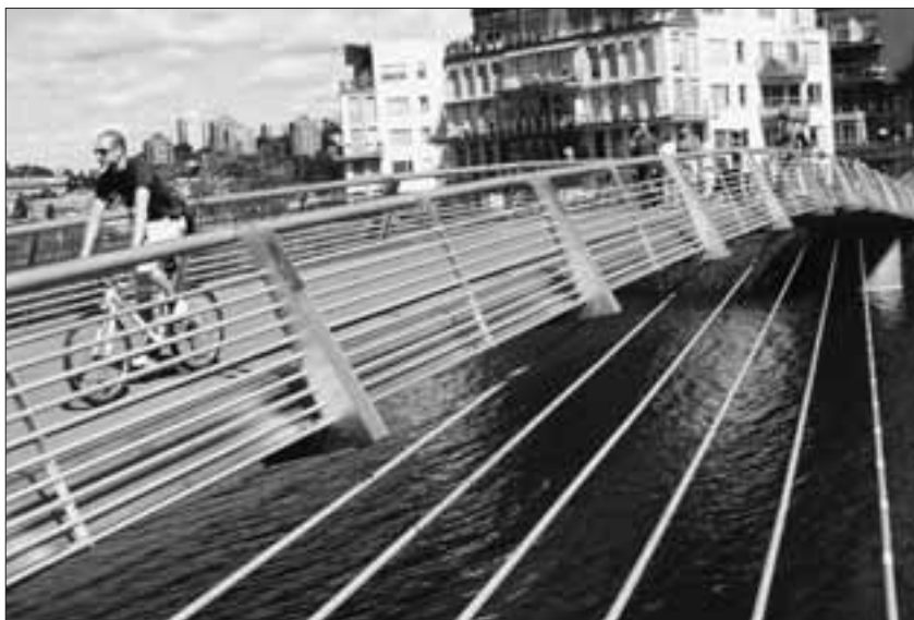
Figure 6.3. Stainless steel bridge in 2205
