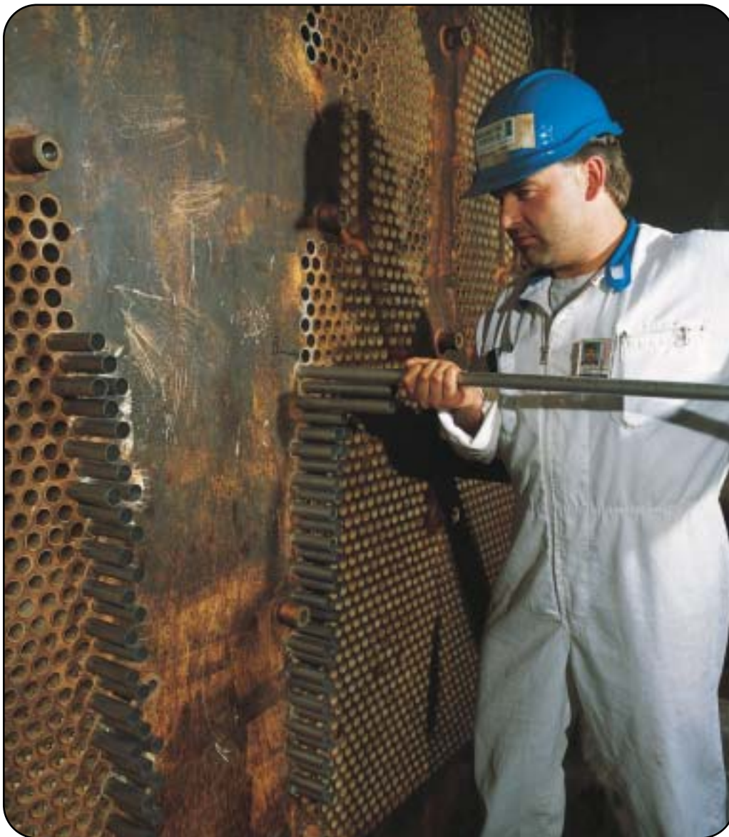
Condenser tubes in 654 SMO ® stainless steel being installed in a nuclear power plant.
