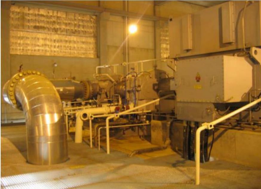
Fig. 20 Explosion Relief panels viewed from inside, note foil covered high density rockwool insulation for sound reduction and fire resistance.
