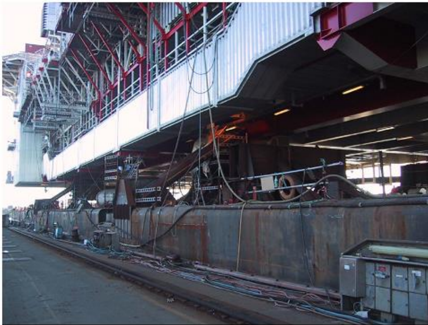
Fig. 29 Gas and condensate platform for 190m water depth ready for load out on a barge, Note Stainless steel fire and explosion proof escape tunnel all along the side (Type 1).
