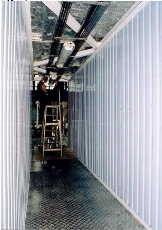
Fig. 30 Inside view of Fixed platform escape tunnel type 1 in Fabrication at Booth Industries in UK: the internal cladding gives an obstruction free escape route: the steelwork of the internal truss can be seen at the top. The top 300mm of the tunnel is service duct.
