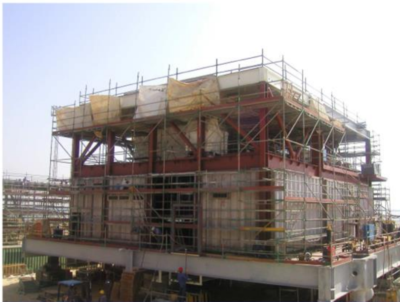
Fig. 10 Stainless steel blastwalls in an offshore module.
