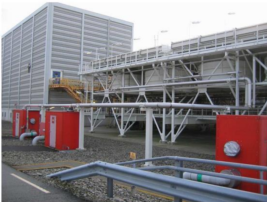
Fig. 23 Kollsnes gas compressor building cladding provides explosion relief for internal explosion (hinged panels for projectile avoidance) and resistance to external explosions and 43dBA sound reduction.
