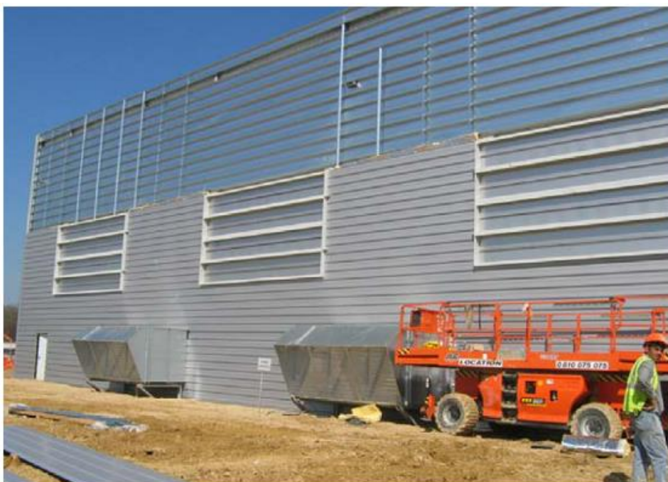
Fig. 19 Stainless steel explosion relief panels installed on a gas compressor building in France.
