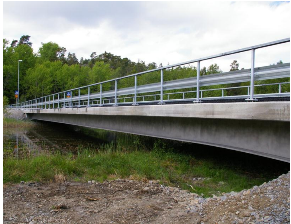
Nynäshamn bridge, Sweden
