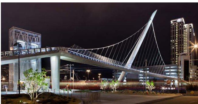
Fig. 7 Harbor Drive Pedestrian Bridge, San Diego, US Photo: Brooke Duthie photography & T.Y. Lin International
